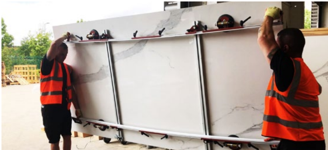
Always use handling frame to manoeuvre slabs
