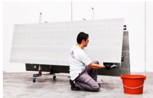
Back-buttering on transport cart
